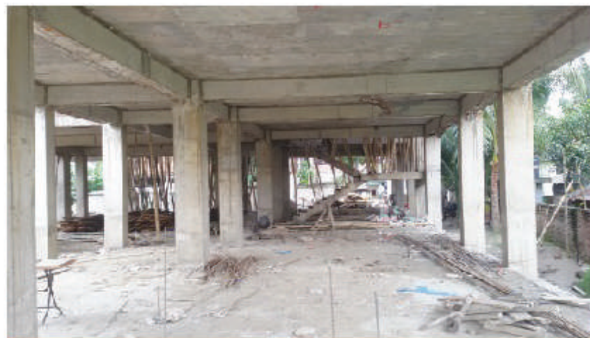
CRP-Manikganj construction in progress
